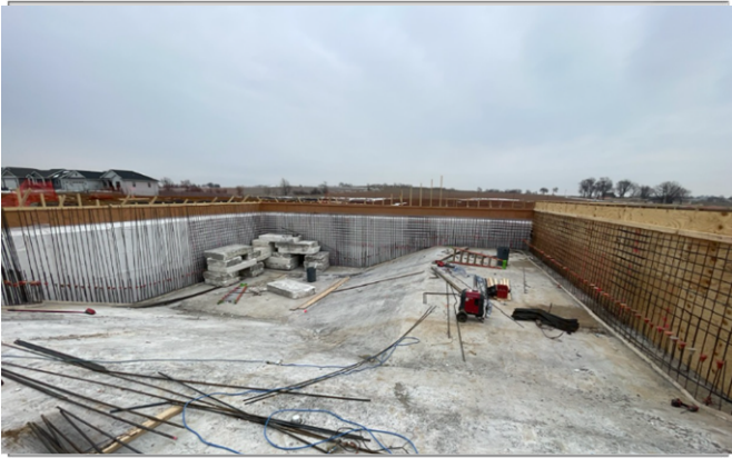
Lap pool wall rebar being installed
