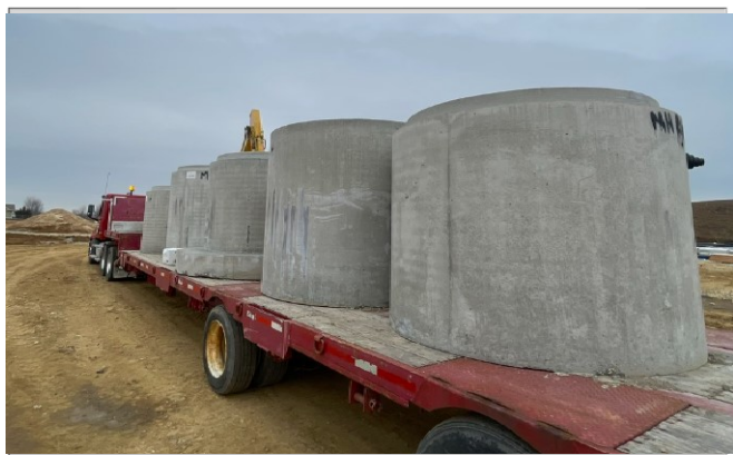
Underdrain structure delivered
