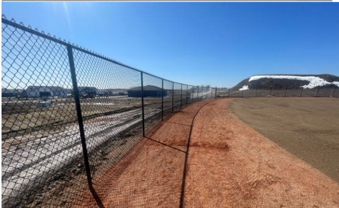
Baseball outfield fence stretched and installed with top rail
