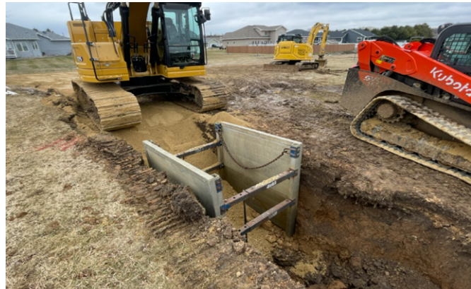
East side water lateral being installed
