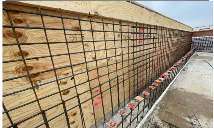
Lap pool wall rebar
